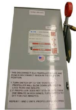
Figure 12. Wind Brake Locked in the ON Position parking the rotor for inspection or maintenance.
