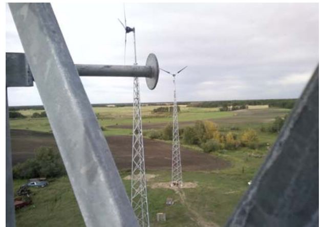
Solar Outpost's installation using Rohn's updated tower design at New Ventera Wind Farm
